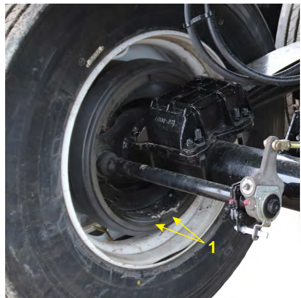
Figure 4-11 – Brake Shoe Lining Inspection
