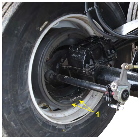
Figure 4-14 – Brake Shoe Lining Inspection
